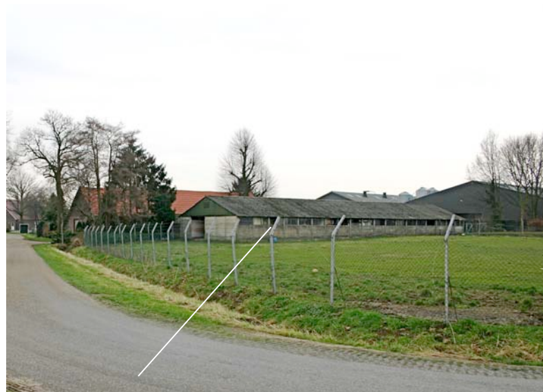
te slopen betonplaten stal
